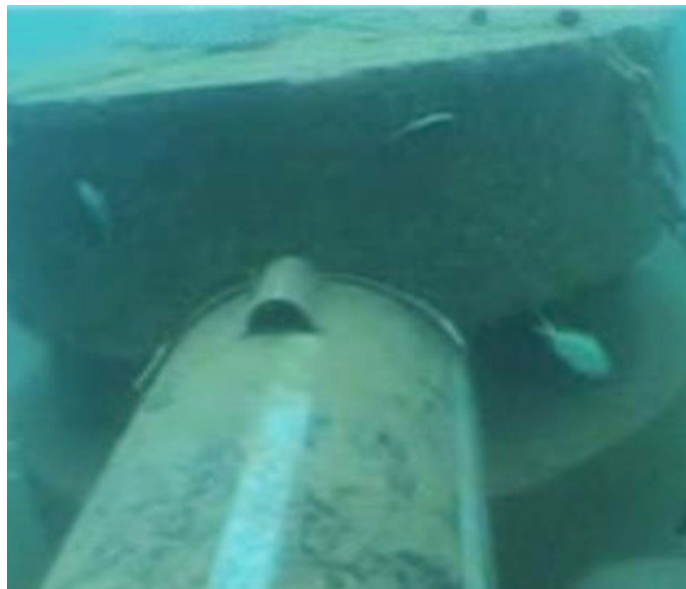
The eco-designed pipe-line after 8 years, in 2017 with coral ecosystem development (lagonia)
