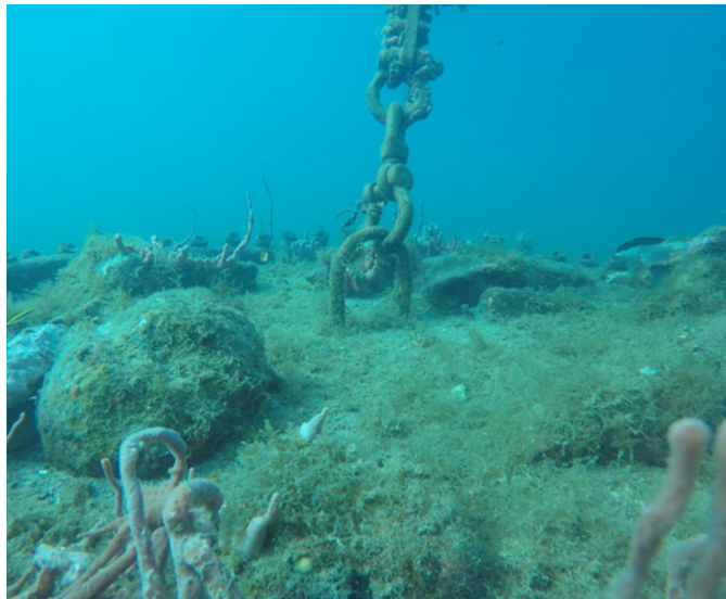
Figure 12: Colonization of an eco-de-signed mooring system 2 years after immersion (Pioch)
