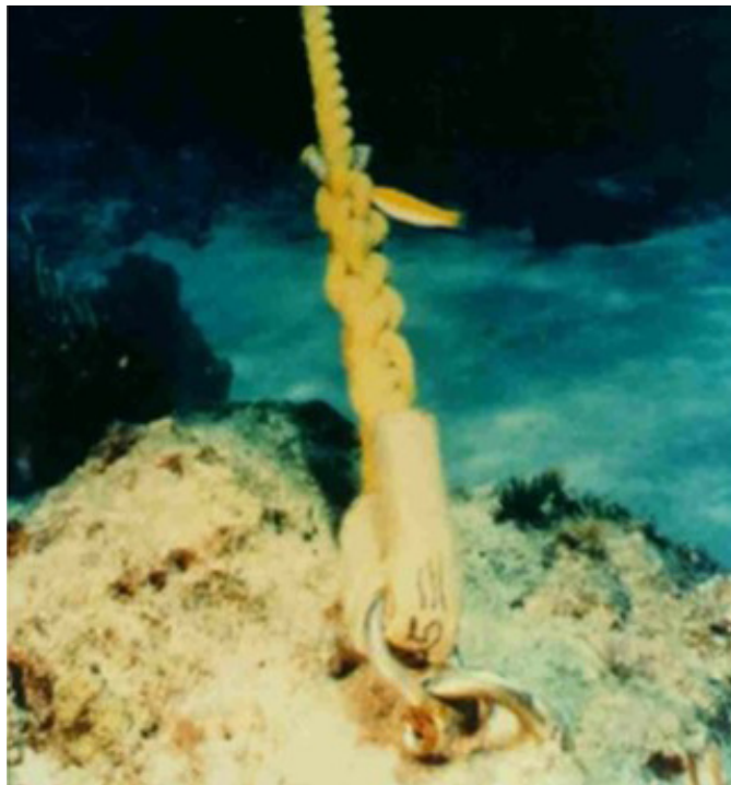
Figure 10: fixed eco-mooring two pictures left eye bolt and right manta ray (padi, 1996; reef relief founders)
